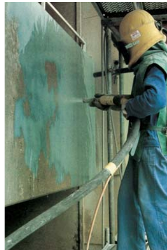
Betonsanierung Concrete refurbishment
